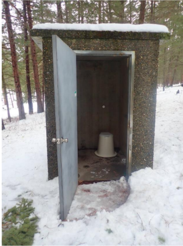
Figure III-2 Example of concrete toilet near Sylvan Lake
